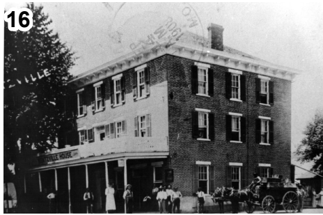
16 1861 (Wentzville House Hotel) - George & Henry Dierker built a three-story frame hotel on the corner of N. Linn Avenue and W. Main (now West Allen). In the same year, it burned down. Six years later, in 1867, the Dierker brothers rebuilt the Wentzville House Hotel. This time the inside and outside walls were of brick, 16 inches thick. In August 15, 1872, George Dierker was granted a saloon license.
