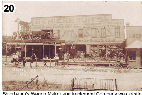
20 Shierbaum's Wagon Maker and Implement Company was located just east of his home and became a landmark of early Wentzville. It had the appearance of an early west settlement business with its huge false front and oversized sign. The Schierbaum Implement Company was sold in the 1920s and became Reuter's Blacksmith shop, which operated until the 1940s, when it was razed and a new building went up to become the American Theater and the Kroger Store. In the 1970s it was sold to Rock n' Roll legend Chuck Berry, who operated it until 1973 when it burned to the ground. Today it is a parking lot.
