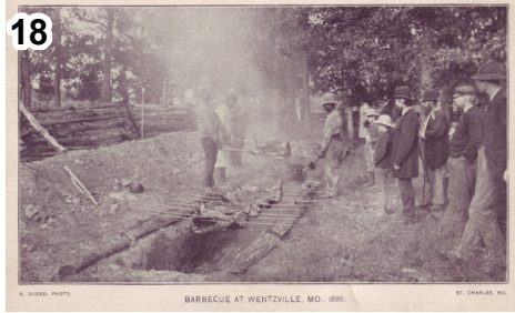
18 Musick Grove today is roughly bordered by Church Street west to Highway 70 and from West Main south to Highway 70. It was owned by Charles E. (C.E.) Musick, and his mansion sat just about where the current MFA is located. C.E. Musick was involved in Wentzville politics from 1890 to 1906, serving five terms as Councilman and Alderman of Ward 1, and in 1904 he was elected Mayor. He hosted many town celebrations on his land, Musick Grove, where townspeople would have huge barbecues for the 4th of July and other events. Wentzville's Craven's Band would play period John Phillips Sousa marches to entertain. Musick Grove is now owned by the Wentzville Community Club, where they hold the weekly flea market and bingo. Musick Grove has been the home of celebrations and entertainment for Wentzville citizens for over a hundred years.
